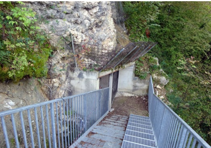
Above: Interior of one of the old galleries opened in the 19th century, currently closed for safety reasons Above: The access staircase to the new Pesciara tunnel, built in 2019
